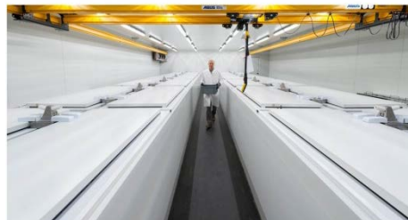
Picture 4. Radix Polaris: two freezing aisles in a cool room. Each aisle consists of twelve sections of one cubic metre each. The resulting 24 m 3 storage space replaces 36 conventional ultrafreezers.
